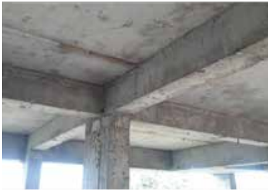
Figure 2. Interior beam-column joint
