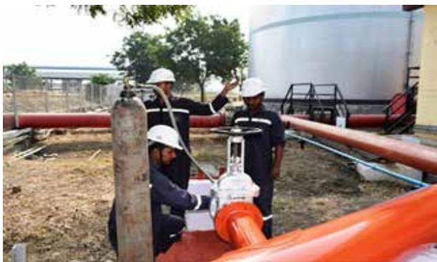
Fig 7. Nitrogen injection in pressurised fire fighting ring network
